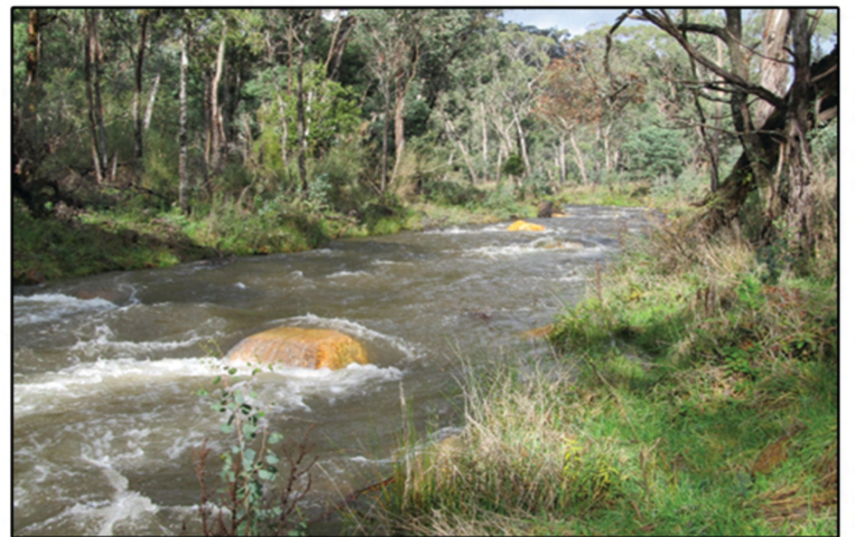
Completed habitat restoration works at Frosty Corner – June 2016
