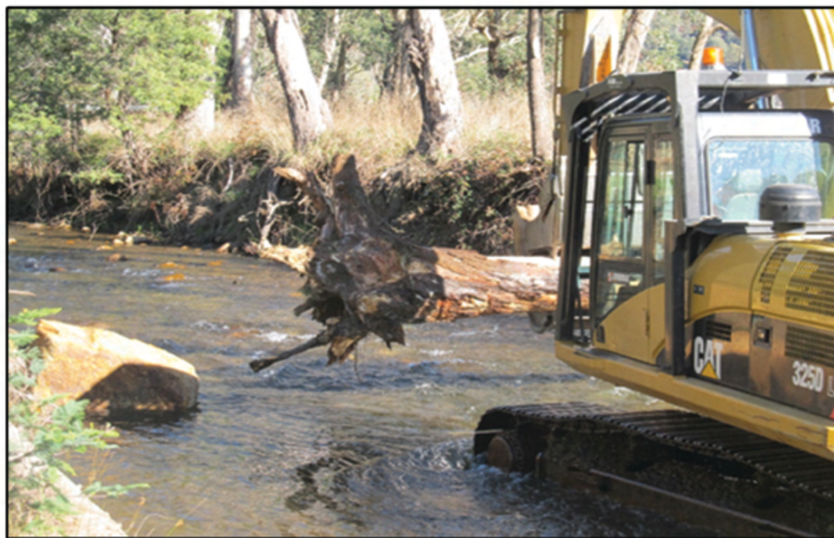
Habitat works on the Ovens River at Frosty Corner, 2015
