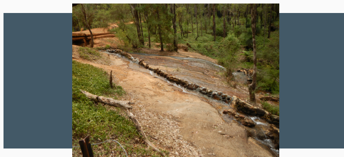
Completed Repairs on the Nanga Brook fish ladder
