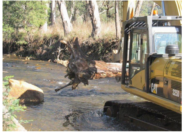
Placing habitat into river
